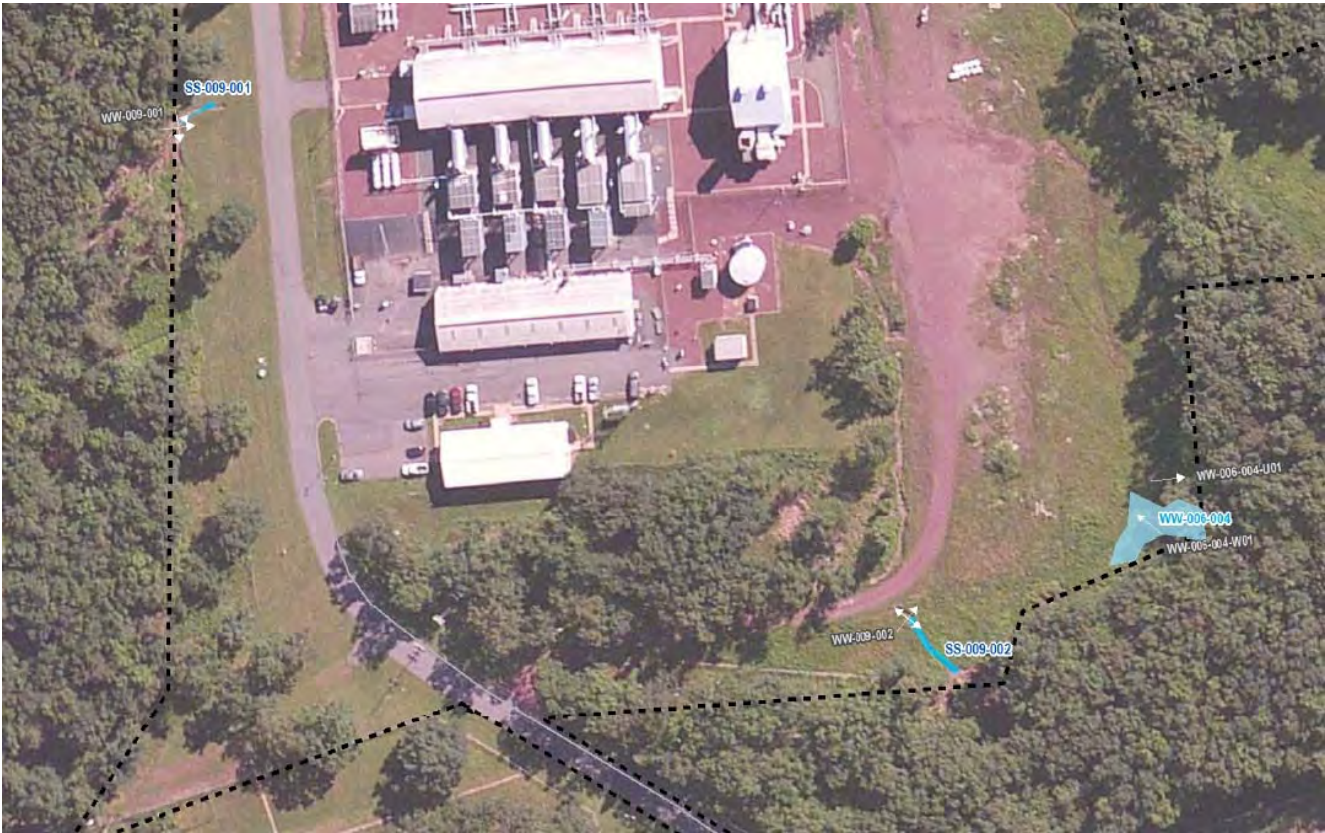
FIGURE 16. Compressor Station 515 at northwest end of proposed Franklin Loop. WW-006-004 and WW-013-001 are shown in the corners of the existing cleared area.
