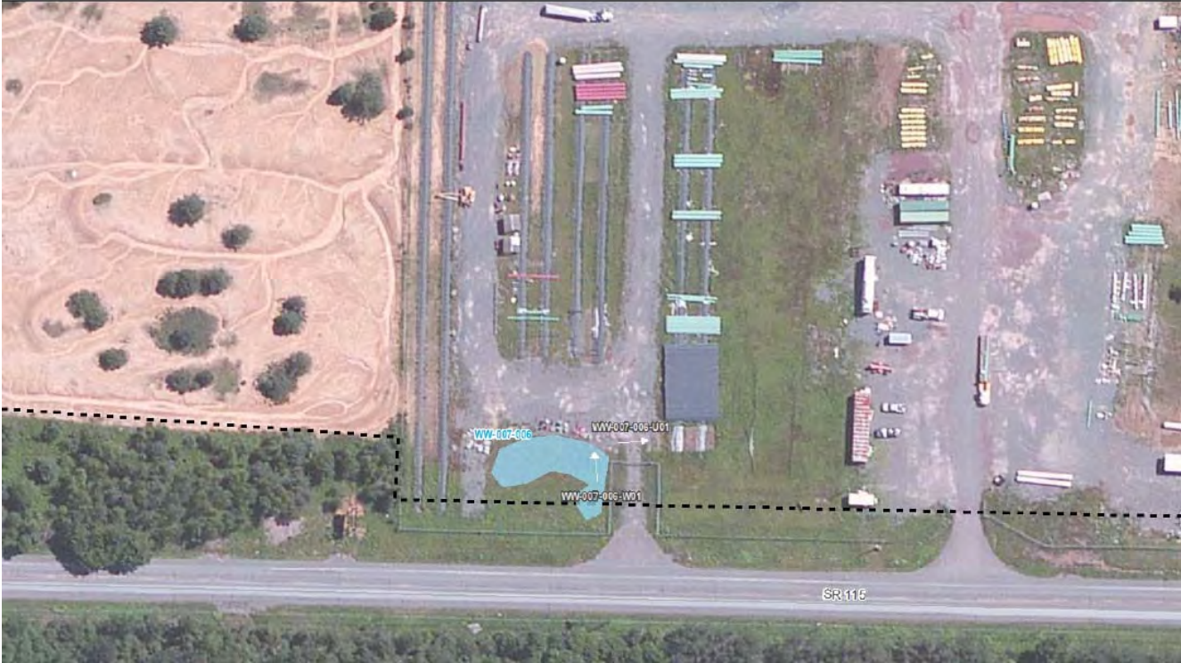
FIGURE 17. WW-007-006 in Mount Effort pipe storage yard beyond southeast end of Franklin Loop.
