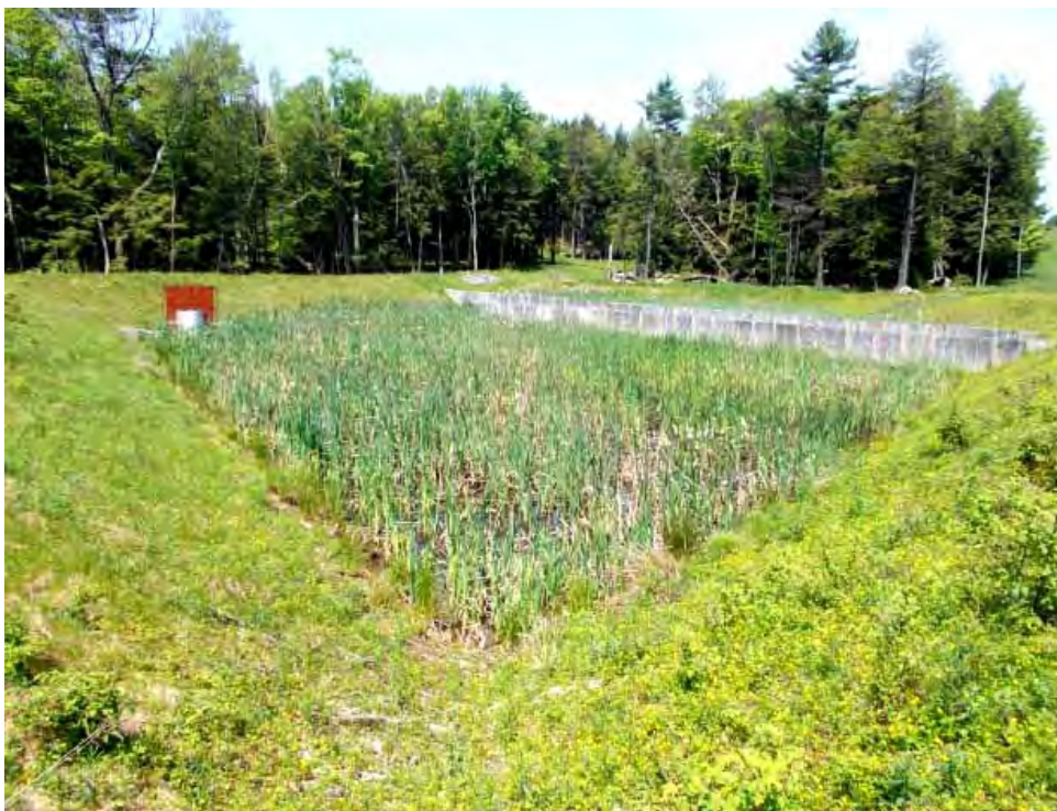
FIGURE 19. WW-001-023 is a manmade stormwater detention basin.
