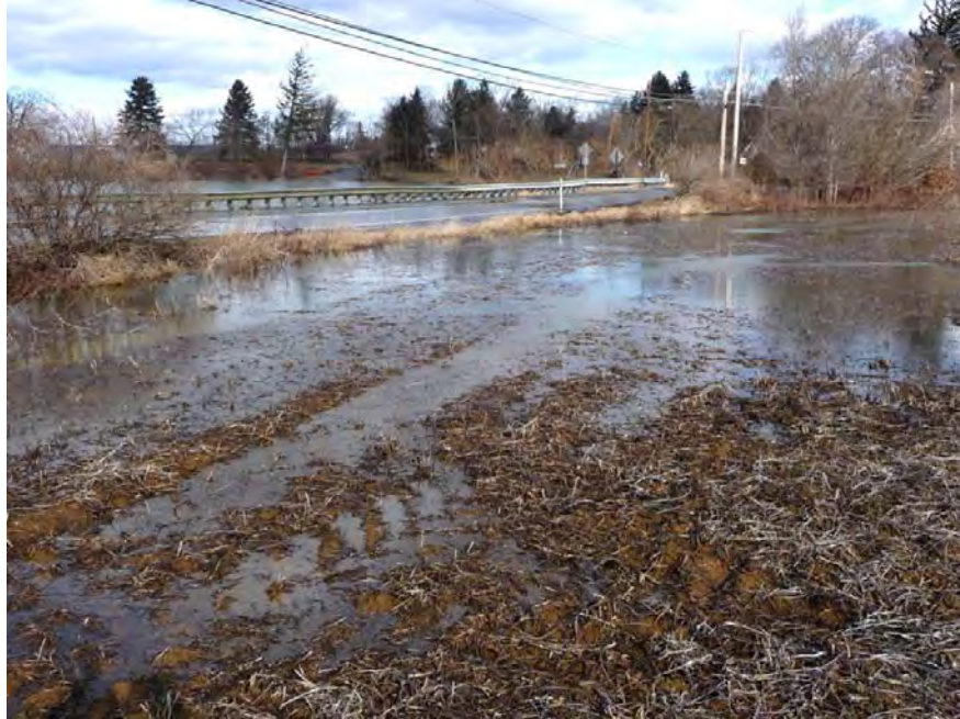
Photo A. View northwest across Green Pond Road, Bethlehem Township, Northampton County, Pennsylvania, 31 January 2013. Typical flow of water over the cartway from Green Pond (background) eastward into Green Pond Marsh during a winter with normal precipitation. Camera is positioned just inside the adjacent farm field.
