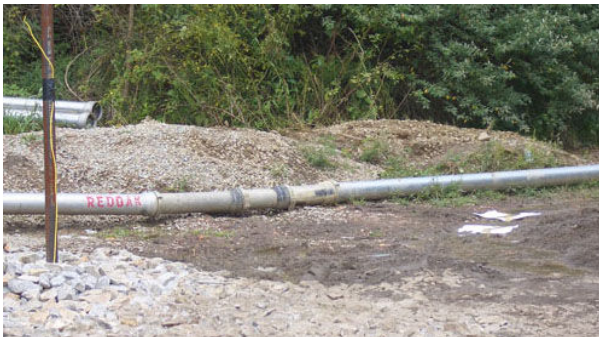
White plastic pipes carry fluids from an impoundment dam
