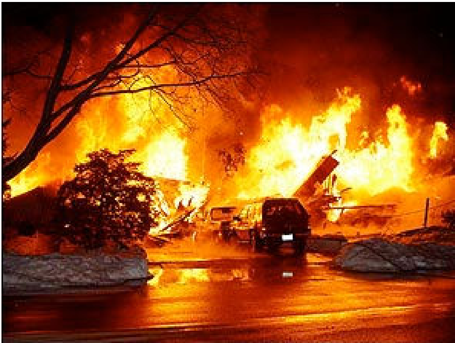
Fire from the buildup of gas from a distribution line leak in a private home.
