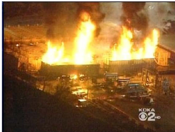
Well pad fire in Avela PA, February 2011.
